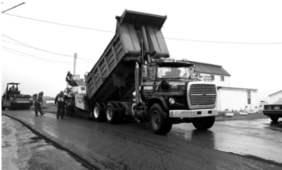
North Side being resurfaced on August 26 th 2005
